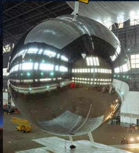
Echo I Satellite 30.5 m sphere L band ca. 1960
